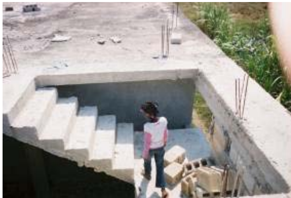
Heroes of Savannah School roof.
