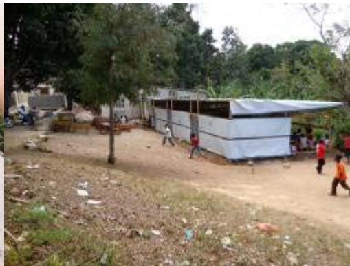
Temporary building at Marechal school.
